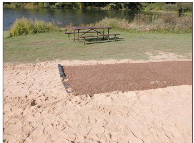
Figure 5—Termination of Soil-Sement portion of beach path. Geotextile fabric visible under completed SEWF surface.
